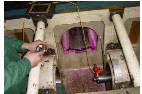
Laser alignment and boring of bearing tunnel
