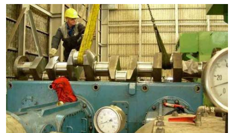
Crankshaft assembled
