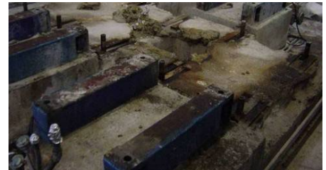
Compressor totally dismantled from the foundation
