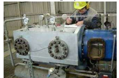
One of four new cylinders installed and tested
