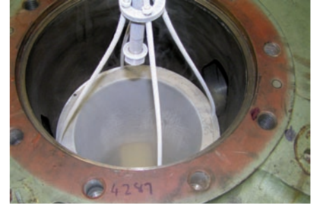
Installation of pre-shrunk liner
